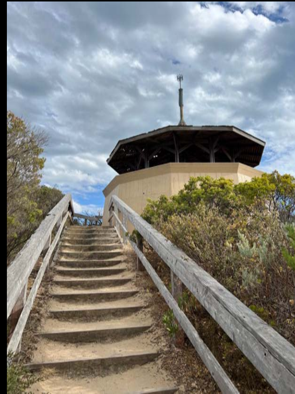
Back Beach Sorrento New Rotunda Coppins Lookout Peter Staughton, architect 1965 drawing, detail NHS Collection
