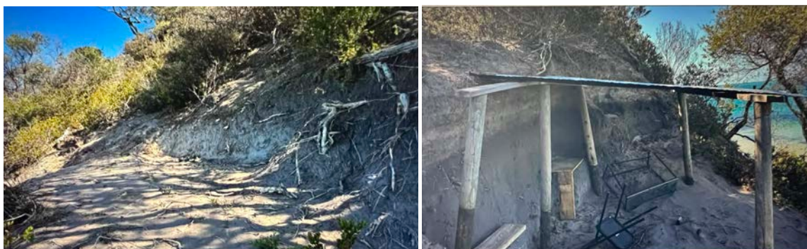
Left: excavation at site 1 near the cliffs; below right: excavation and building assemblage at site 2 near the cliffs. Reinstatement and restoration is extremely difficult, particularly on the cliff edges.
