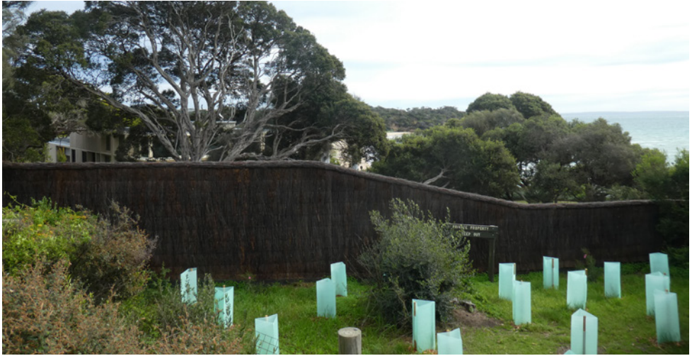
New fence on the Eastern Sister, erected under VicSmart. It no longer permits the public to view Sullivan Bay and the Western Sister. Photo Ursula de Jong
