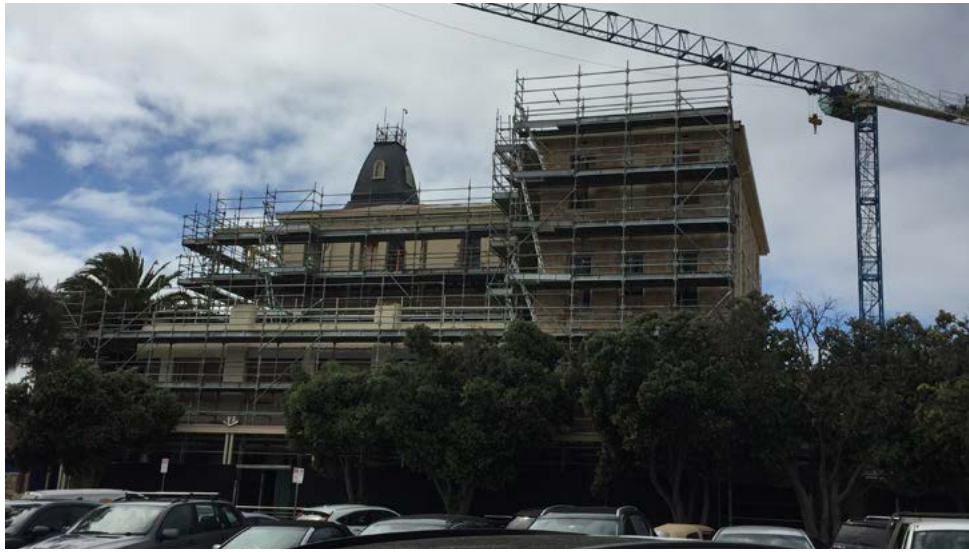
Continental Hotel, under scaffolding, December 2019. Photo: Ursula de Jong
